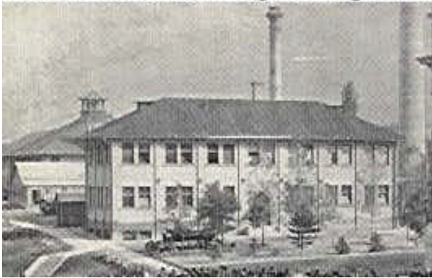
Plate 7 Mechanical Bldg. looking north
